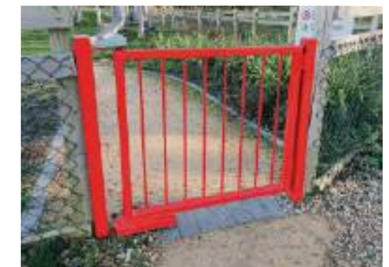
APSSTOP SHOWN IN GATE
